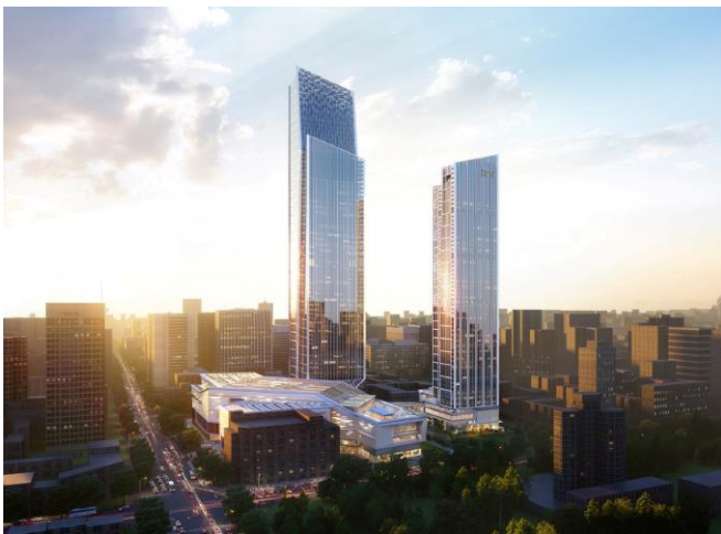
Grand Hyatt Kunming, with a gross floor area of 49,560 square meters, will occupy the first 26 floors of the hotel and residential tower (right). The hotel will become a prestigious addition to Hang Lung's mixed-use Spring City 66 development in Kunming. (Remarks: the photo is an artist's impression for reference only)
