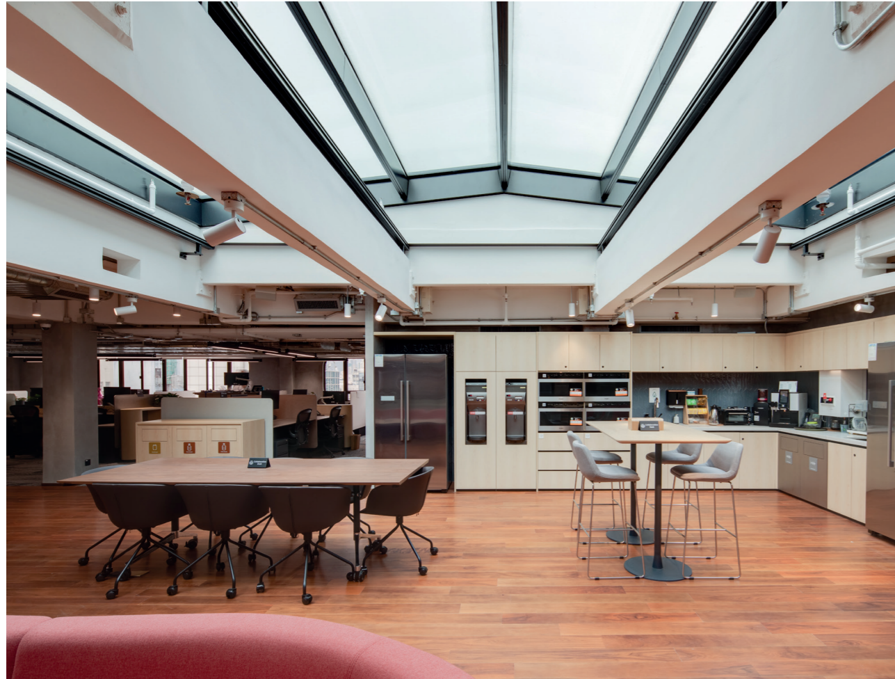
家乐坊办公室加设天窗，引入自然光 Newly opened skylights in Gala Place office introduce abundant natural light
