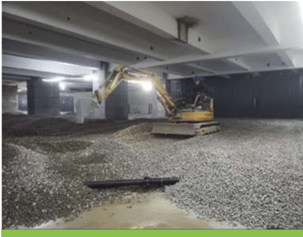
Back filling the recycled aggregate in Westlake 66 basement
