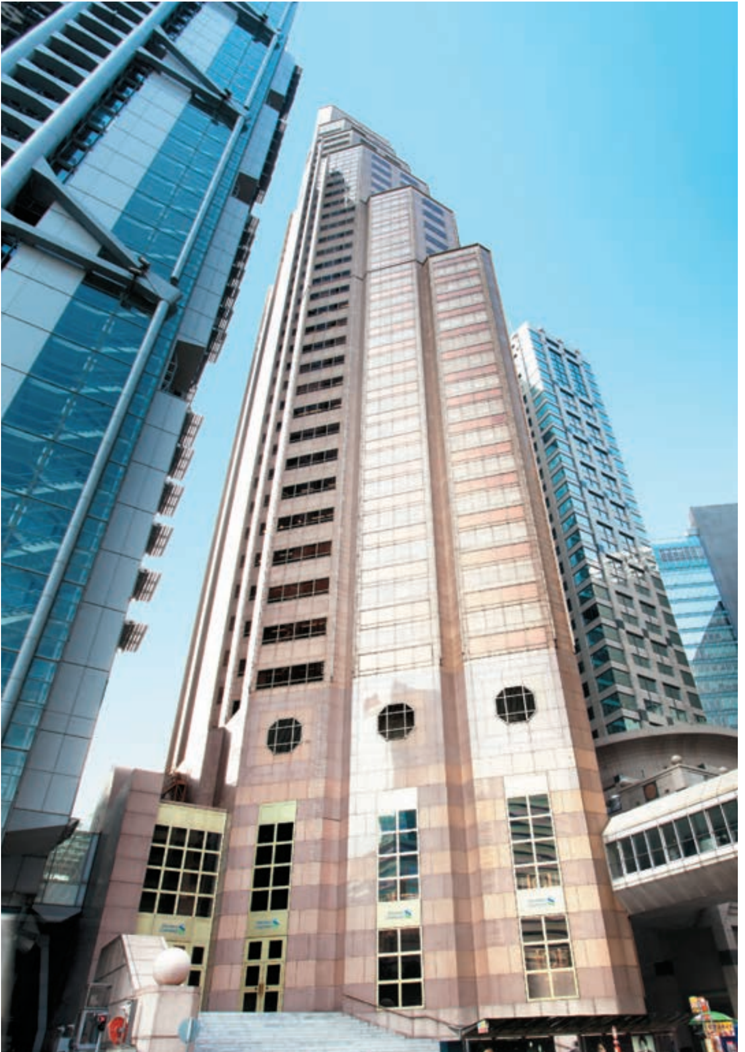
Standard Chartered Bank Building, Hong Kong
